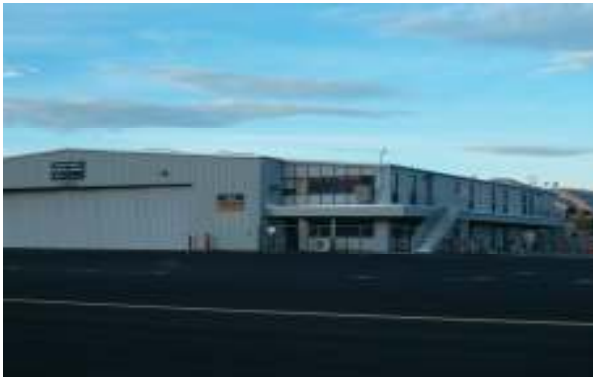
Remodeled Operations and Maintenance Building U42
